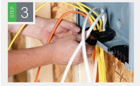
Snap on the Qwik-Grip shield when all circuits are installed
